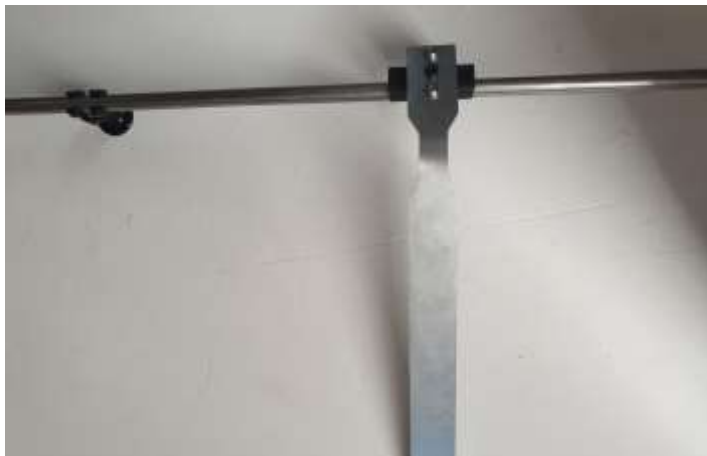
Angled drilling tool placed at pipe
