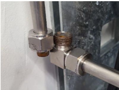
Demount the high-pressure pipe. Demount the by-pass hose
